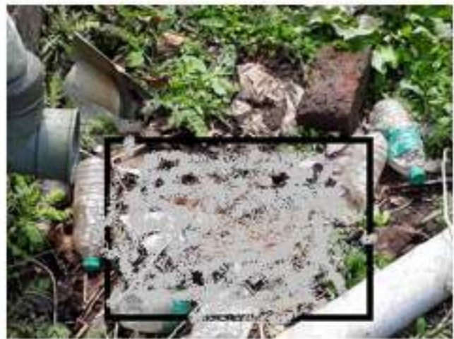
Toilet outlet pipe of the school is in a broken condition resulting feces contamination on ground
